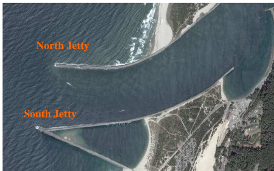
Figure 2. Douglas County South Jetty - proposed site for the Wave and Tidal Energy Project (Image obtained from Google Earth)
