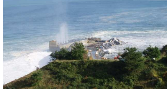
Figure 1: Mutriku plant in construction. The picture shows columns of water flowing through the holes of the power take-off system.
